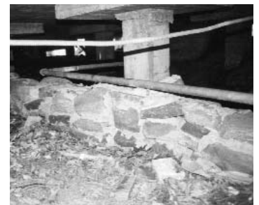
(TOP LEFT) Fig. 76: Oblique aerial view of Ojibway Hotel showing south wing, probably before 1970. (TOP RIGHT) Fig. 77: 1907 photo possibly showing part of south addition, Ojibway Hotel. (ABOVE) Fig. 78: Stone foundation wall of original south addition, under present kitchen wing.
