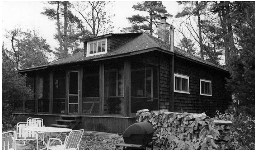
(TOP) Fig. 149: North elevation, Oakwood. (MIDDLE) Fig. 150: North-west corner, Oakwood. (BOTTOM Left) Fig. 151: Plan, Oakwood. (BOTTOM Left) Fig. 152: Interior, Oakwood.
