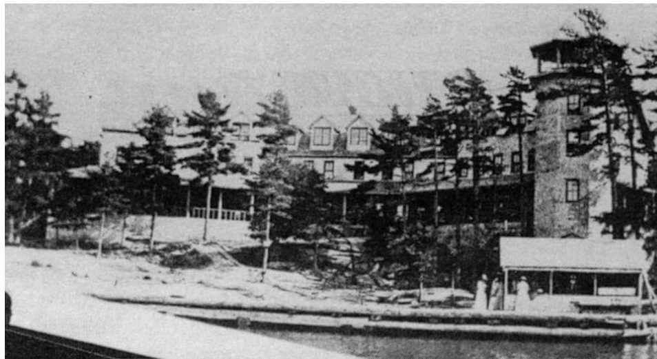
Fig. 19: Same elevation, probably 1912. Note that chimney 2 (serving verandah fireplace) does not yet exist.
