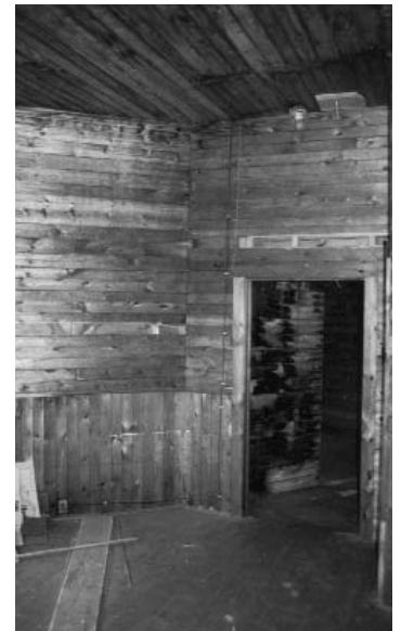
(TOP) Fig. 92: Lounge before electricity, probably 1910 - 1920. Note wallboard and battens, log columns, furniture and gas lamps. (ABOVE LEFT) Fig. 93: Doors in Café, note chair rail on wall with horizontal boards above and vertical boards below. (ABOVE) Fig. 94: Third floor tower room with similar chair rail and board configuration. (BOTTOM) Fig. 95: Dining room, with chair rail, vertical boarding below, unfinished above.
