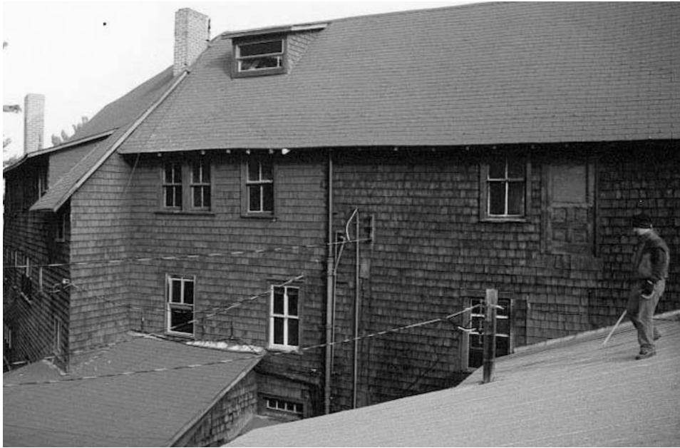
(TOP) Fig. 79: South elevation of Ojibway Hotel, central section.
